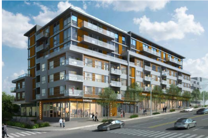
Figure 2: Revised Development as Viewed from Corner of Renfrew Street and 10th Avenue
