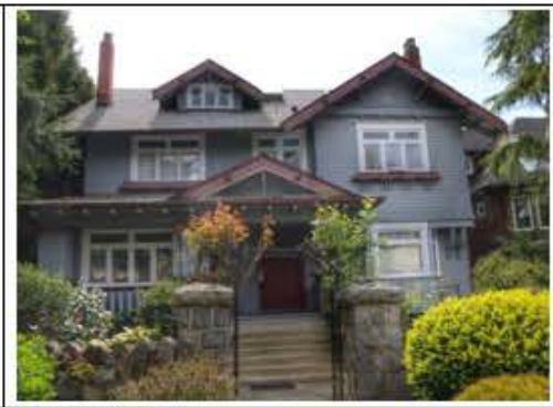
2536 W. 2nd Ave Built 1912 Next door to proposed development
