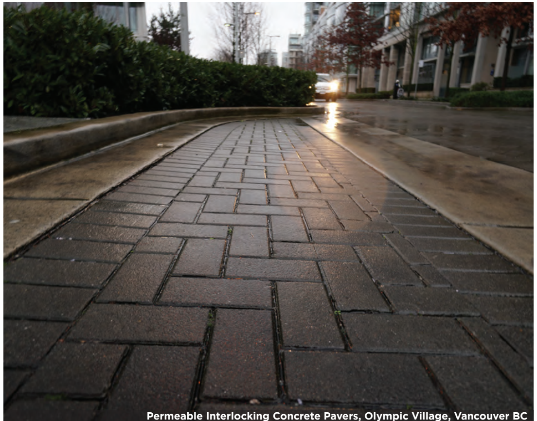
Permeable Interlocking Concrete Pavers, Olympic Village, Vancouver BC
