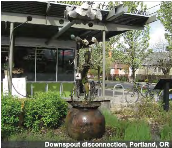
Downspout disconnection, Portland, OR
