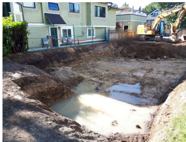
Figure 8: Groundwater encountered during excavation
