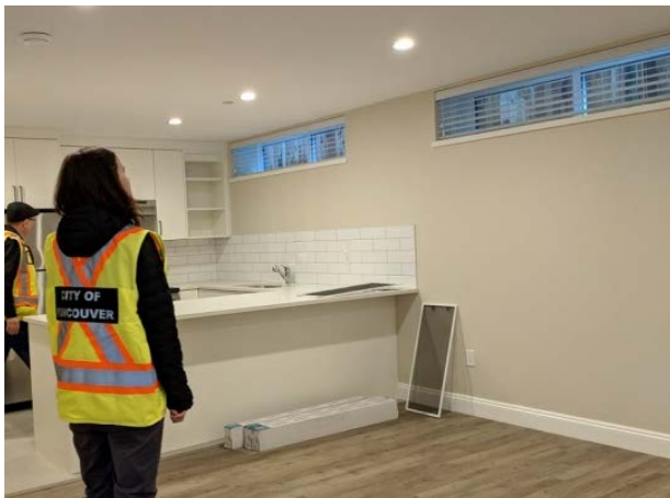
Figures 1 & 2: Deep basement with small windows (left), below grade windows with light well (right)
