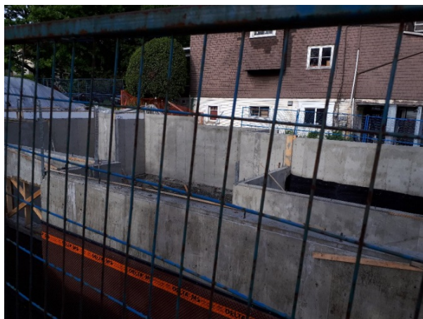
Figure 7: Extensive excavation, decreased tree retention and reduced permeability
