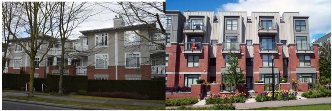
Figure 12: Varied rooflines on multiple dwellings
