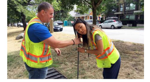
(of students) will go house-to-house in Kitsilano and Riley Park, using a device that uses sound to detect the presence of a leak. They'll listen to the curb stop valve, which is where a home connects to the city's water-main network. We'll let the homeowners know about any leaks found, and ensure they are fixed. If the first trial is successful, this could become a regular summer program.
