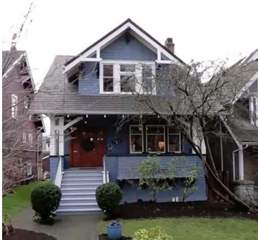
Front (north) façade of house
