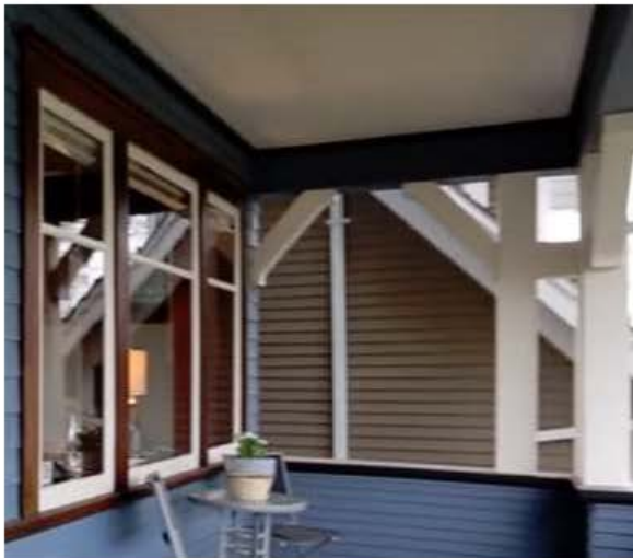
Figure 38: Exterior storm sashes at living room windows
