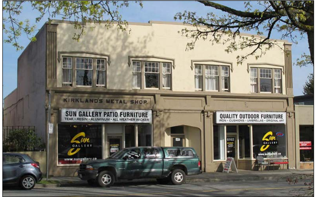
Photo: West Façade of Kirkland's Metal Shop
