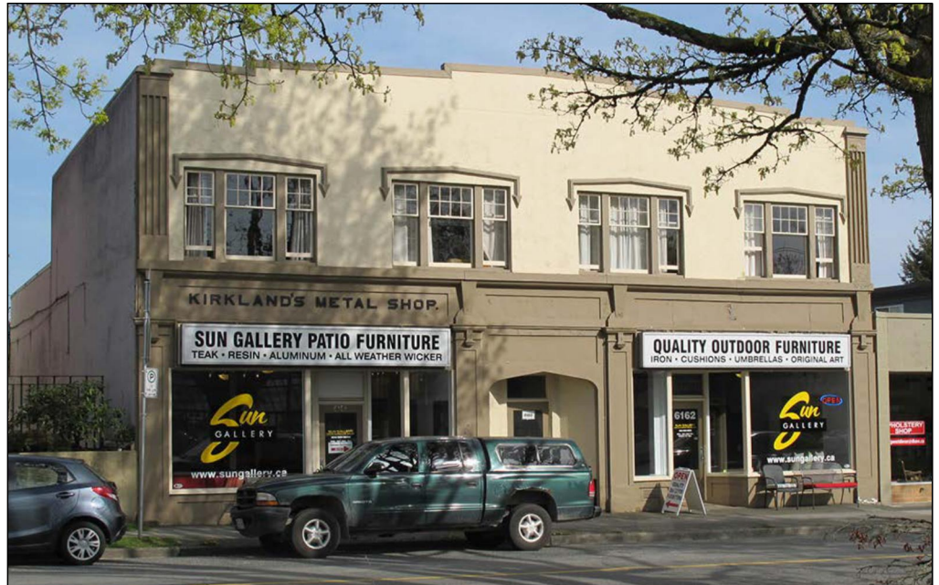
Photo: West Façade of Kirkland's Metal Shop
