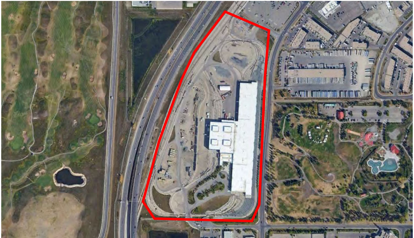
Figure 7-2: Oliver Bowen LRT Maintenance Facility, Calgary. Approximately 13 hectares with 2,800 linear metres of storage track. Stores 108 x 26m Siemens LRT vehicles. Site has abundant amounts of unused space.
