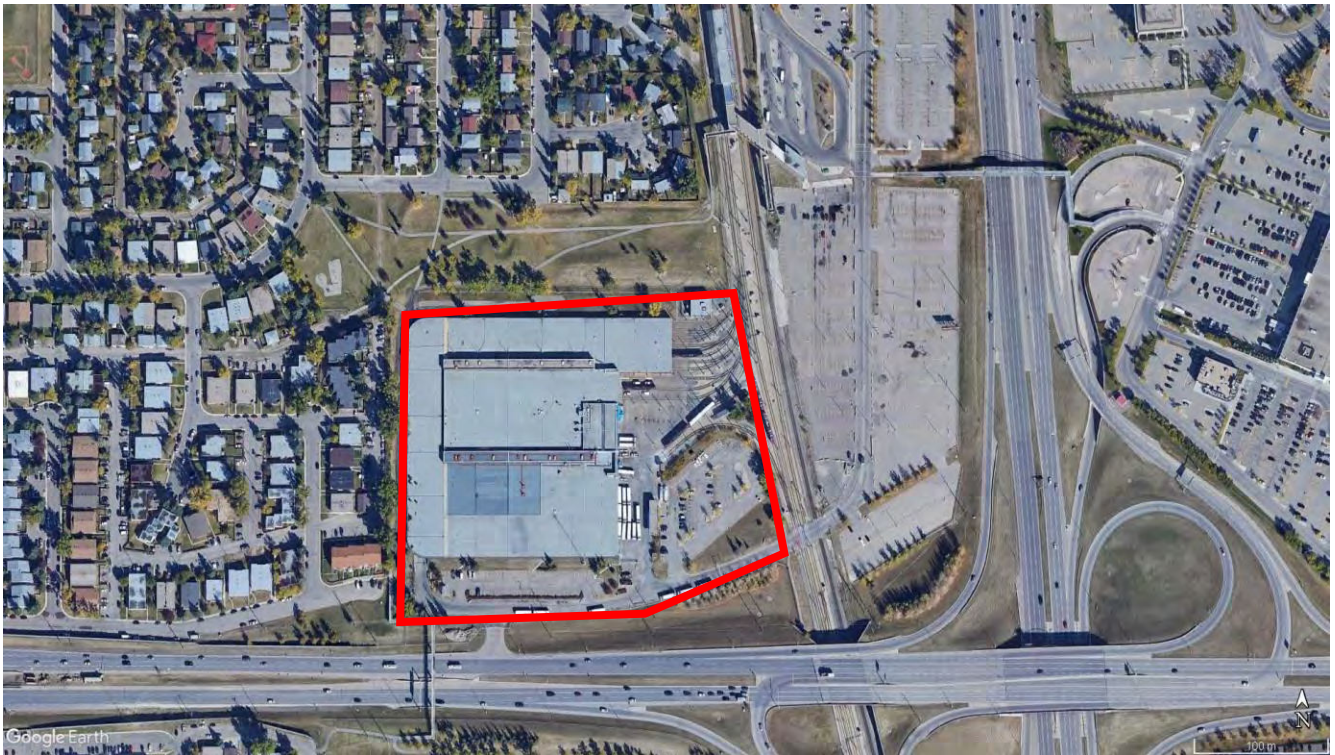
Figure 7-4: Anderson LRT and Bus Garage, Calgary. Approximately 6 hectares (effective LRT area approximately 3.5 hectares). Stores approximately 54 x 26m LRT vehicles on 1,400 linear metres of track. Efficient site use with limited turnaround track functionality.
