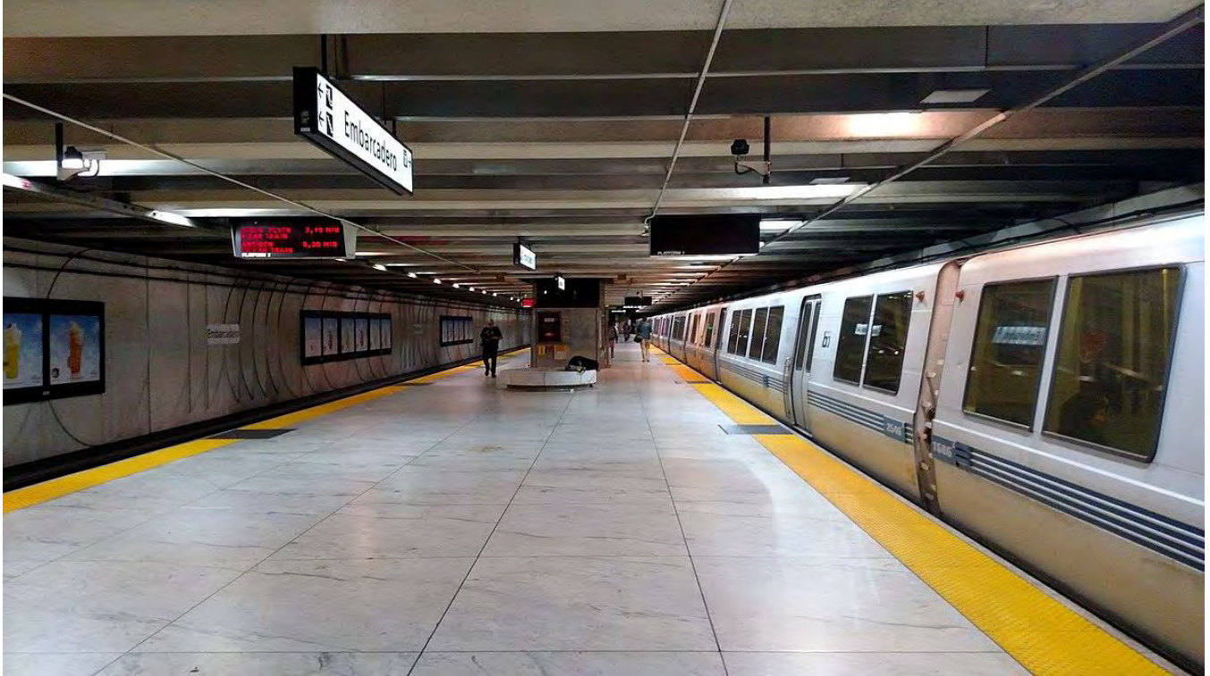
Figure 12-1: Existing Embarcadero Station Platform
