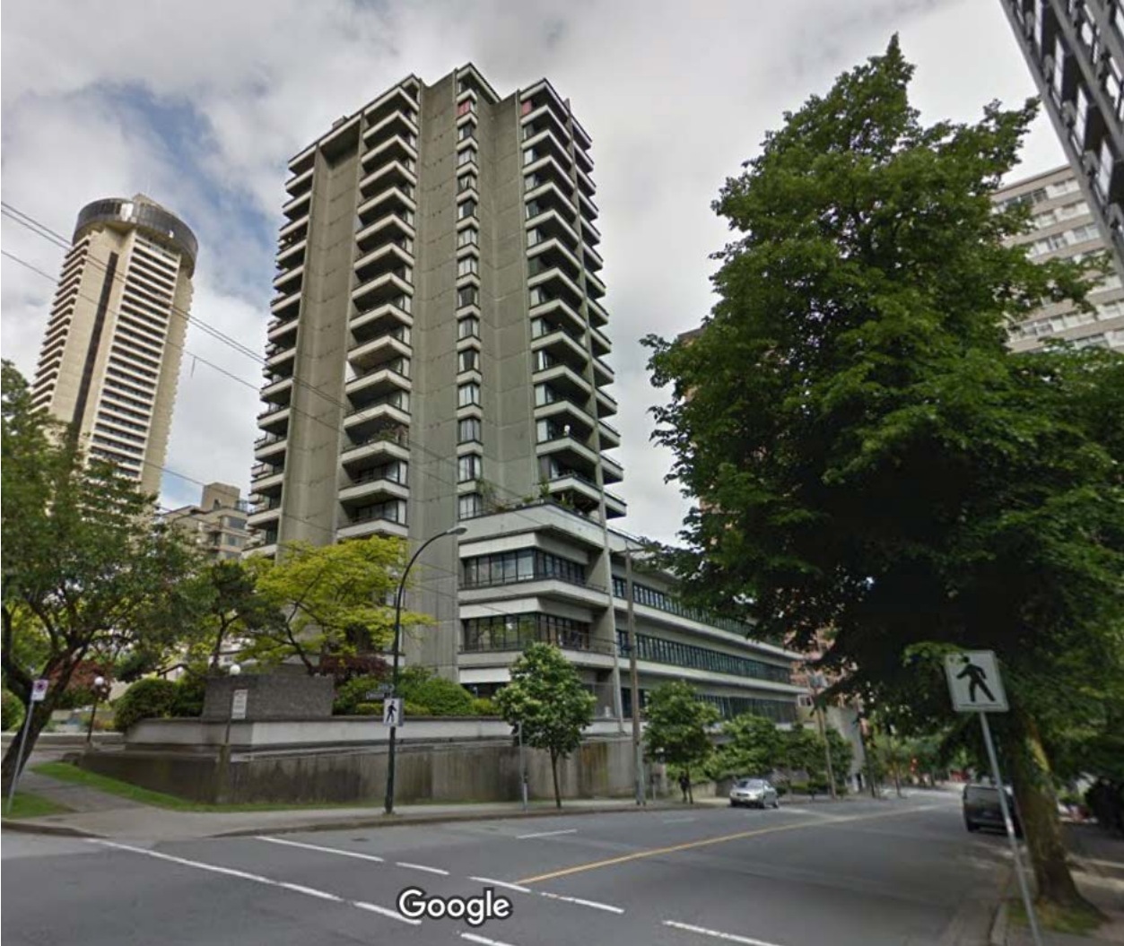
1444 Alberni Street Image Source: Google Maps
