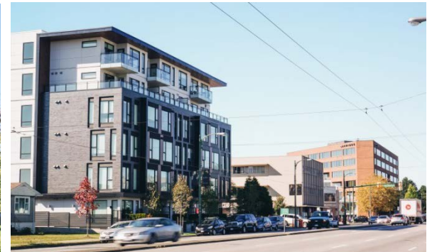
458-476 West 41st Avenue - 50 secured market rental units
