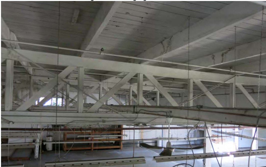
Figure 5 - Hanging Roof Truss
