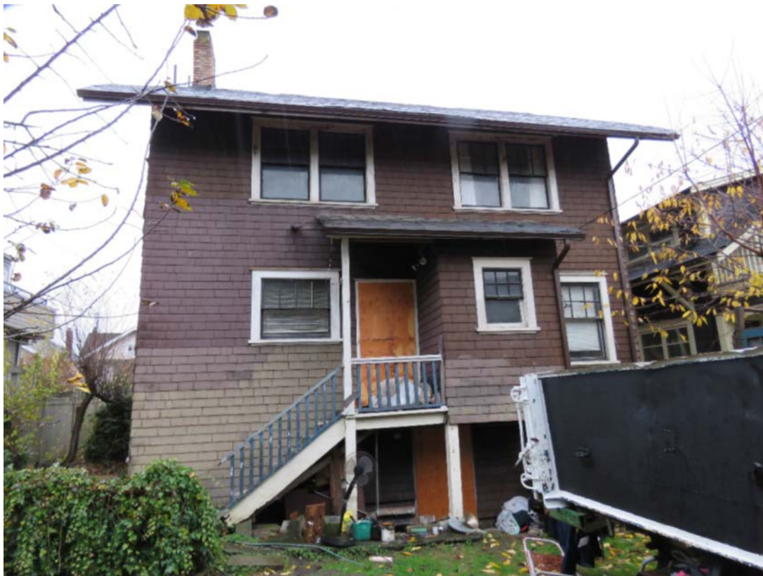
2425 West 5th Avenue - Front Elevation
