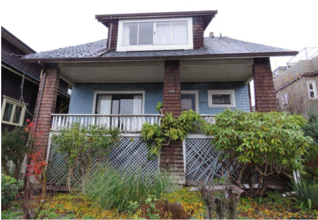
2425 West 5th Avenue - Front Elevation
