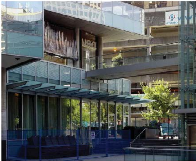
Existing Open Bridge and Restaurant Terrace View (from the pedestrian pathway)
