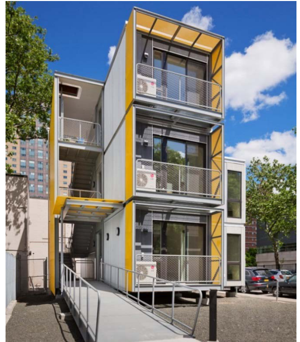
Buildings should be sited close to grade to minimize ramps and railings (Urban Post-disaster Housing, US) Photo: TBD
