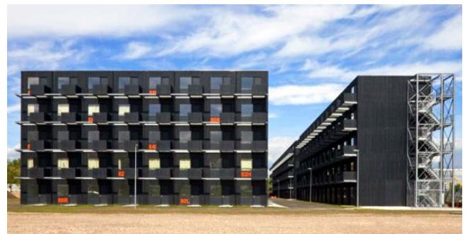
Balconies add depth and visual interest to a modular façade (Zuidezeeweg Modular Student Housing, SZ) Photo: TBD
