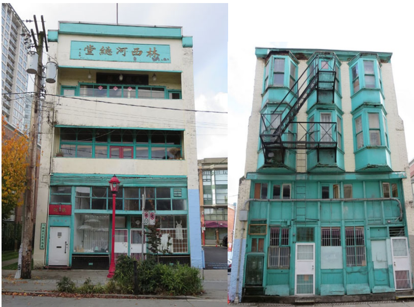
Figure 2. Lim Sai Hor Association Building - Carrall Street and Shanghai Alley facades - current condition
