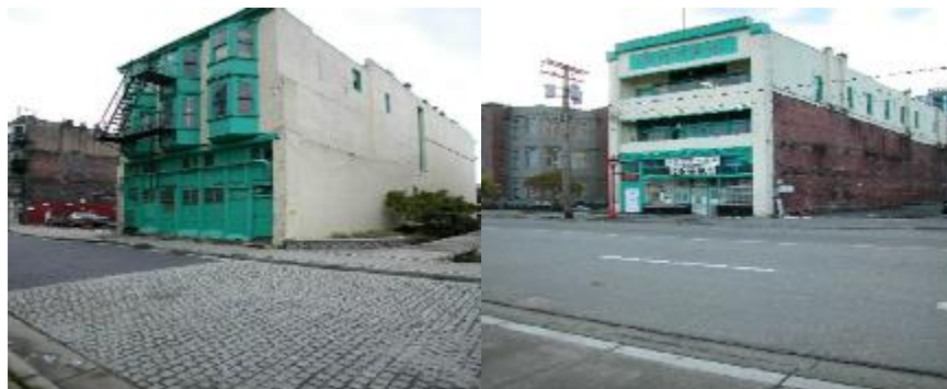
Rear facade and side
