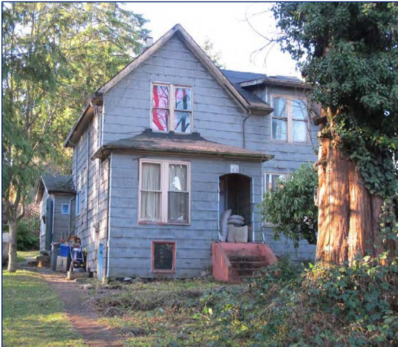
3365 Commercial Drive: Existing Location and Condition
