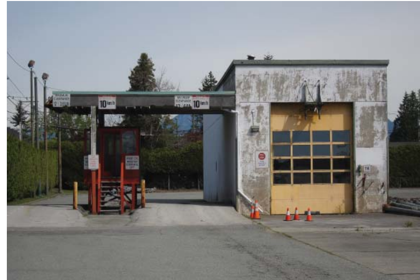
Photo of wash rack at northwest corner of OTC Site (April 2014)
