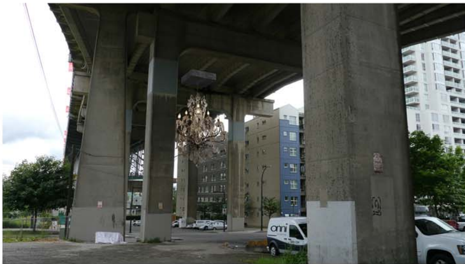
View toward southwest under Granville Bridge
