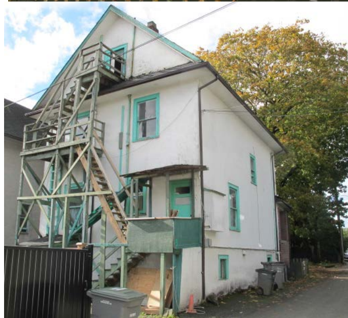
Photos 1 and 2 : Front (West) at Top and Rear (East) at Bottom (circa 2015)
