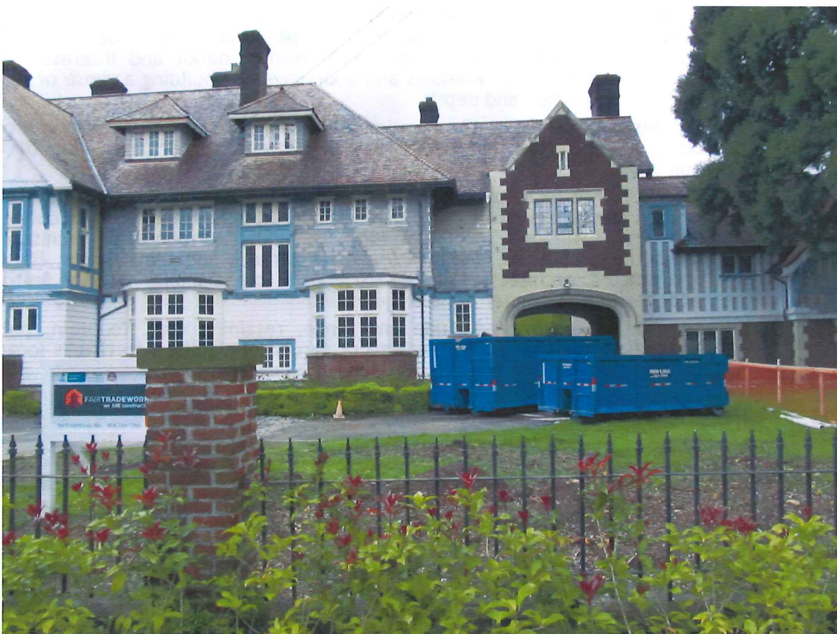
Above: Rosemary, 3689 Selkirk Street, 2015. View from the front yard of the ongoing refurbishment of the exterior cladding.
