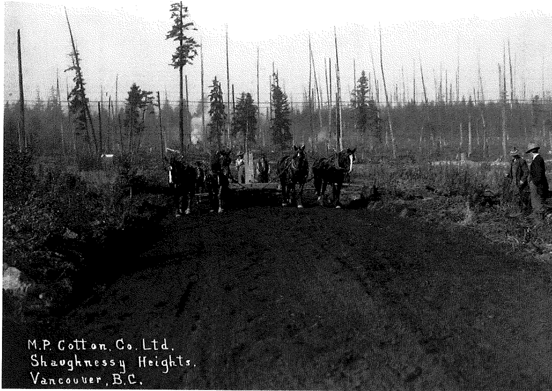
M.P. Cotton Co. Ltd. [engineers and general contractors] road clearing in Shaughnessy Heights, 1911 [City of Vancouver Archives; Above: 677-251; Below: Dist P20]
