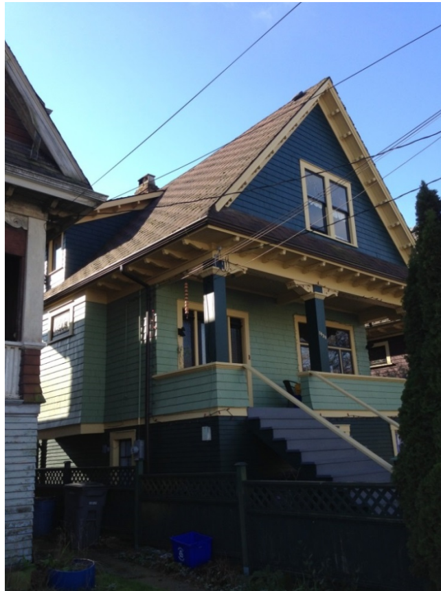
1938 Ferndale Street - Margaret and Joseph Dick House, front and east side
