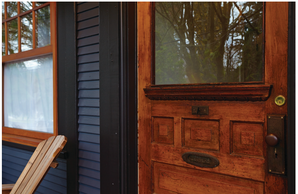
Above: The original windows of this character home had been replaced with aluminum frame windows. In restoring the home, the owner chose to install new, custom wood frame windows that fit with the home's heritage character.
