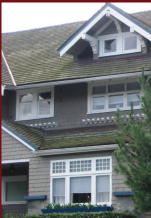
Existing windows do not need to be replaced.
