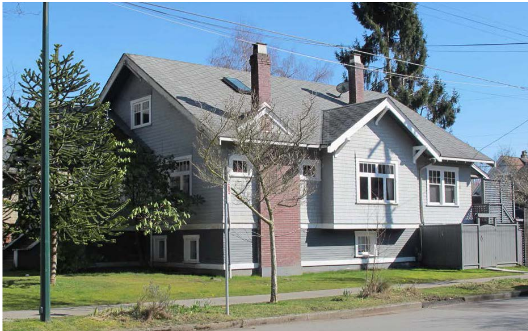
Photo 2: 1010 East 21 st Avenue (West Side, Looking East) circa 2014
