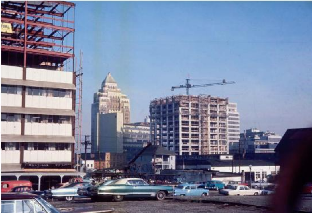
Bentall Centre under construction, February 1966, CVA 780-18
