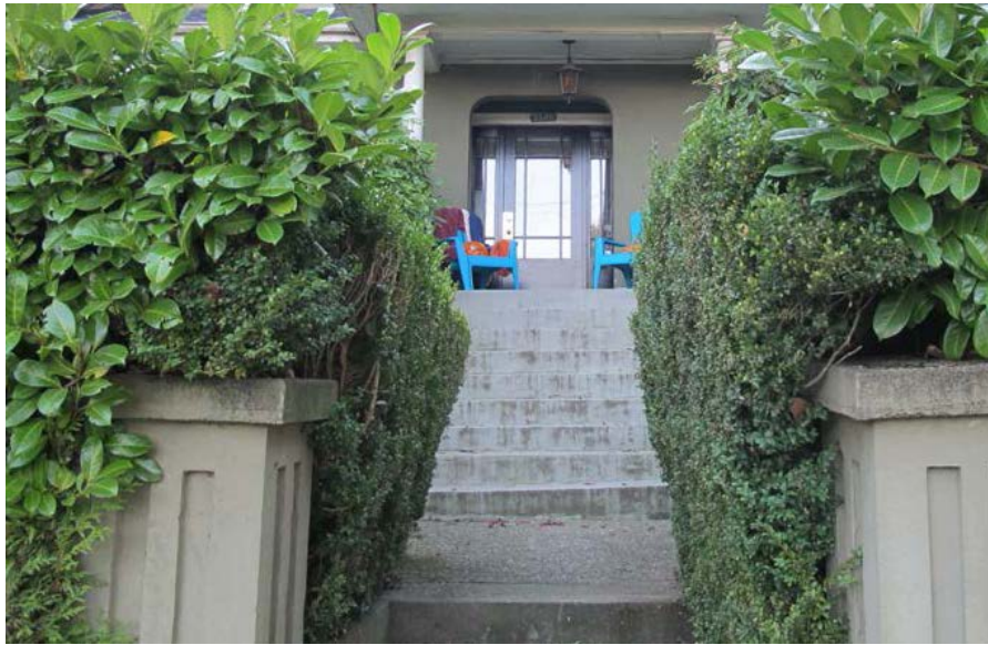
Photo 5: The front Entrance of the Evans Residence
