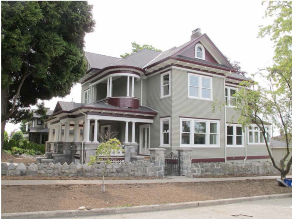
The Ramsay Residence circa 2014 (Rehabilitation Completed)
