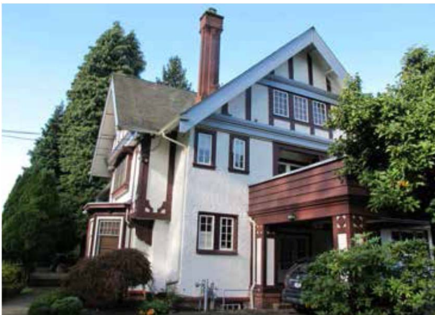
East elevation with porte-cochere
