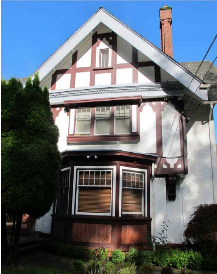
Details of front elevation: Stucco cladding, half timbering, dentils, "herringbone" brick pattern in lower section of bay window
