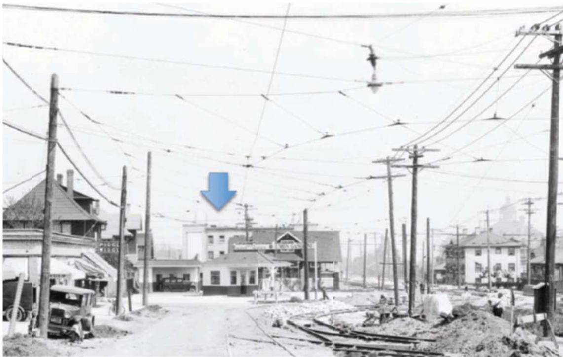
Photo 3: The Van Arsdel in 1929, as indicated by the arrow, looking south from Oak Street and East 17 th Avenue. The apartment building on the far right between the telephone poles still exists (see Map 2 in Appendix A).
