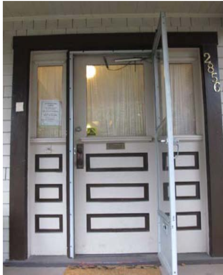
Photo 3: Original front door assembly (2013)
