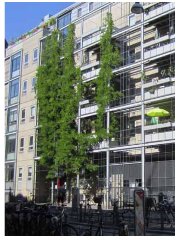
Detail of facade at Cambie
