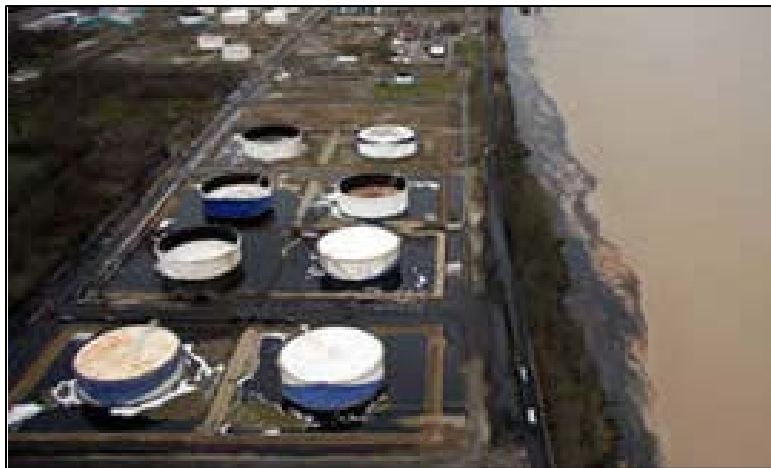
Aerial view of the Ambès oil depot and the slick, following a tank rupture. France 12/04/07 (Source Cedre)
