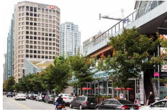
Office, hotel, retail and restaurants on Alberni Street in the Central Business District.
