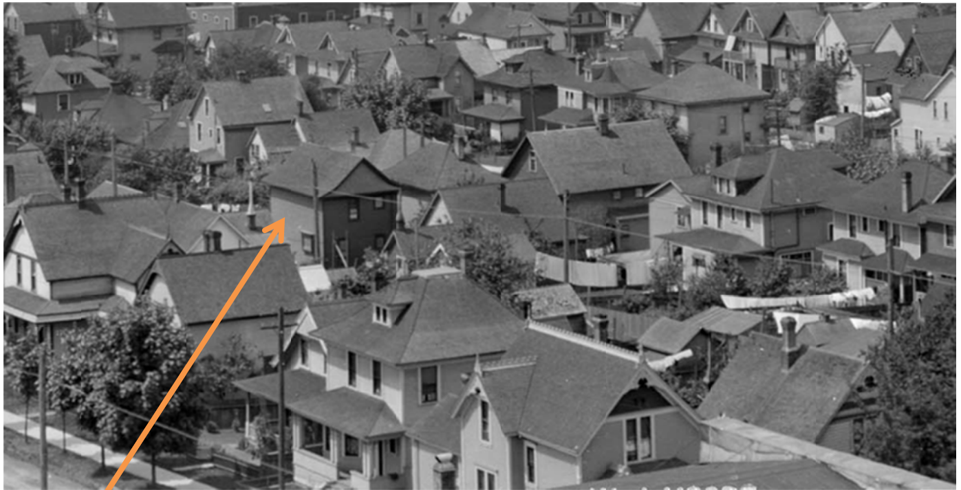
Photo 1: 2322 Ontario Street, circa 1913, looking north-west
