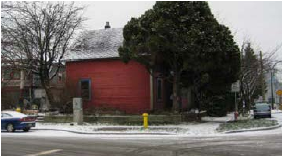
Photo 5: View of the south side of 445 Vernon Drive, looking north (2011)
