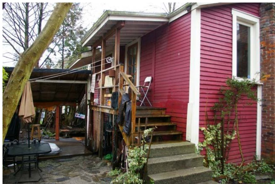
Photo 9: The 1903 House, 431 Vernon Drive (2011) looking north, on-site
