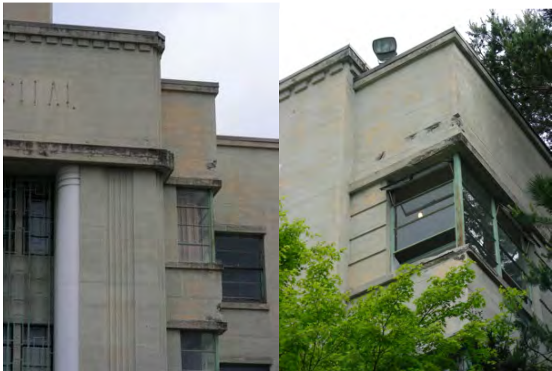
Figures 2 and 3 Detail of concrete elements, corner window with damage concrete hood
