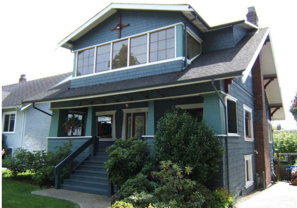
3350 West 37 th Avenue - Black House - North (Front) and West Elevations
