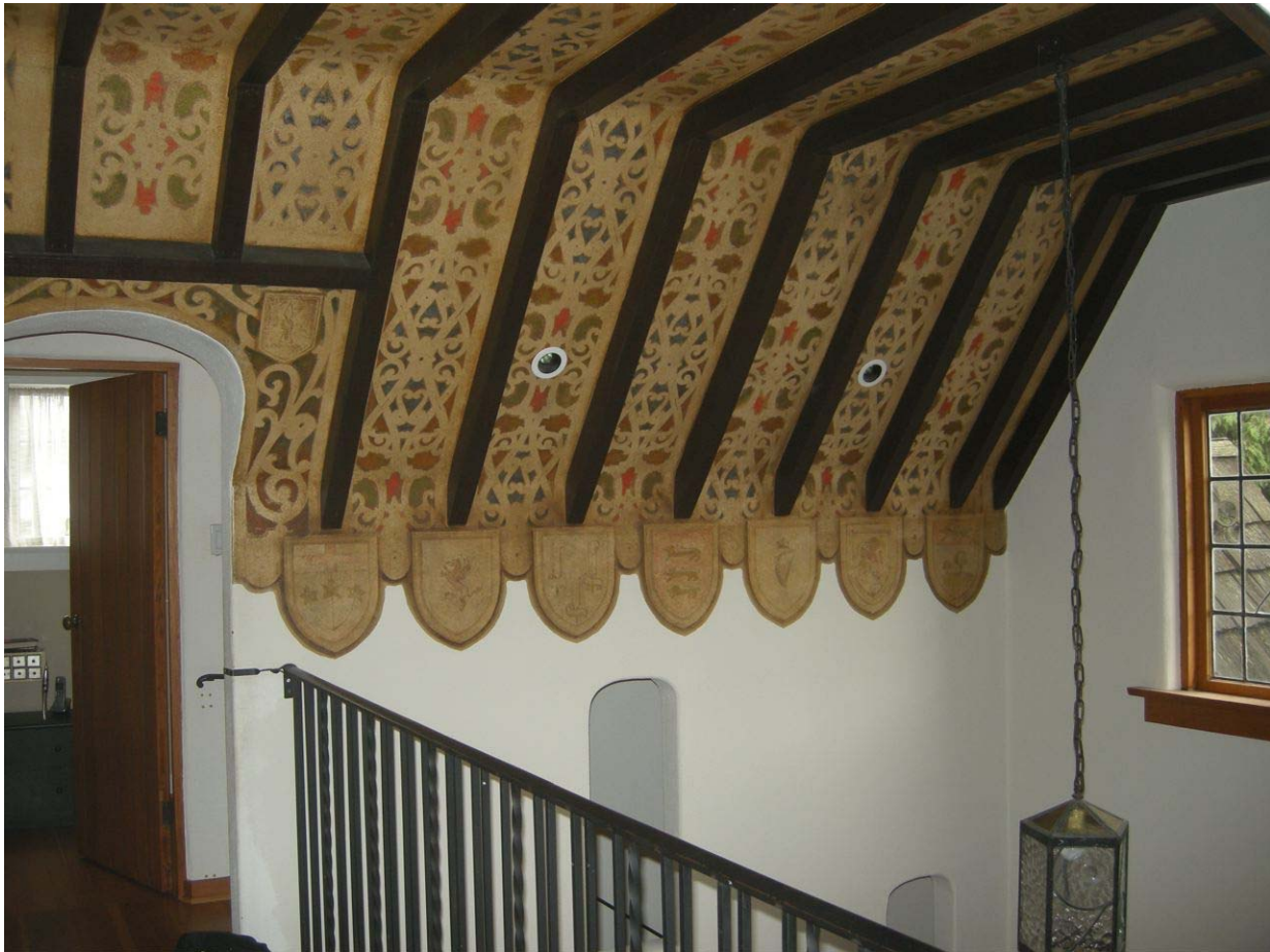
Photo 6: The ceiling today (circa 2011)
