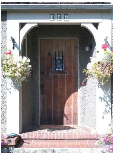
Photo 4: Close-up of the wooden-plank entrance door (circa 2011)
