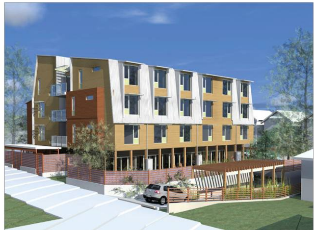
4 View along Lane and entry into underground parking looking northeast
