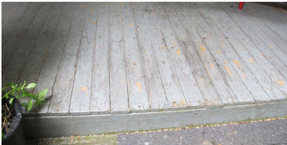
Photo 2: The original porch floor appears to still exist, which is rare. The proposal is to retain and repair, sand, and repaint the original wood planking.
