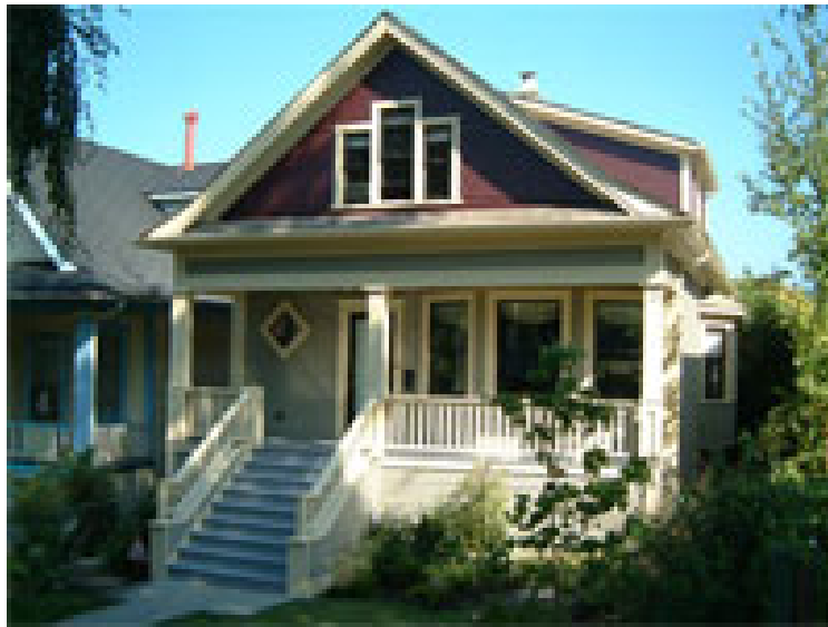
Photo 5: 1943 East 4 th Avenue. This house had been modified in the past in a similar manner to 'The Lee Residence', including the enclosure of the front porch. It was restored to its original condition based on photos provided by the families of early residents of the house, similar to 'The Lee Residence' proposal. In 2009 the owner was awarded a Heritage Award of Merit by the City for the rehabilitation of the heritage building, which was added to the Vancouver Heritage Register in 2009
