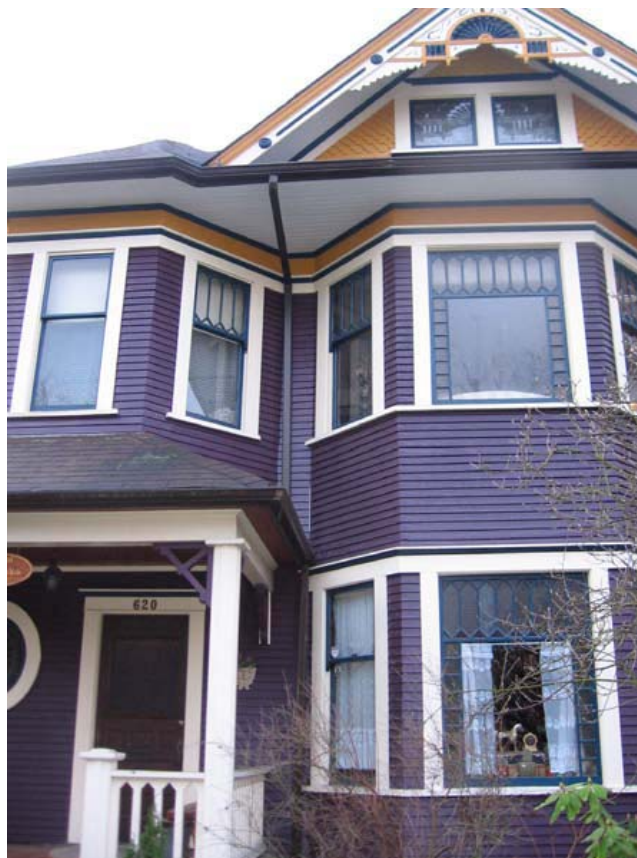
Close Up of the Front of 'The Bezzasso House' (2010)
