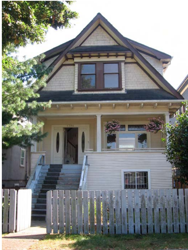
Front of 'The Tibb House' at 1784 East 14 th Avenue
