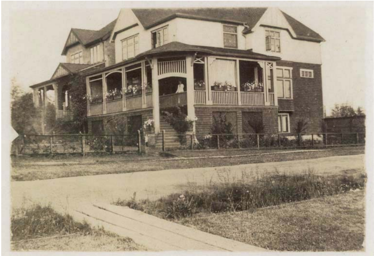
Figure 1. Historic photo of Kydd Residence (circa 1919)
