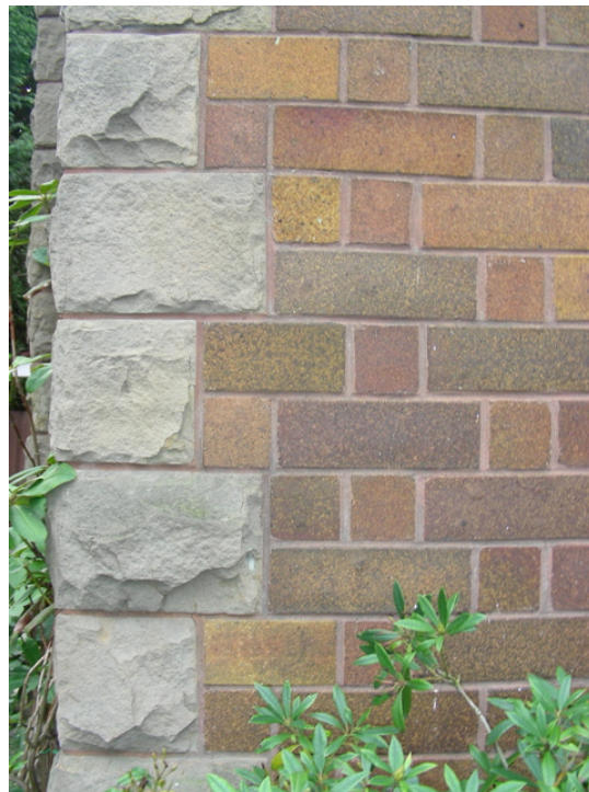
Photo 4: Close up of Masonry Detail
