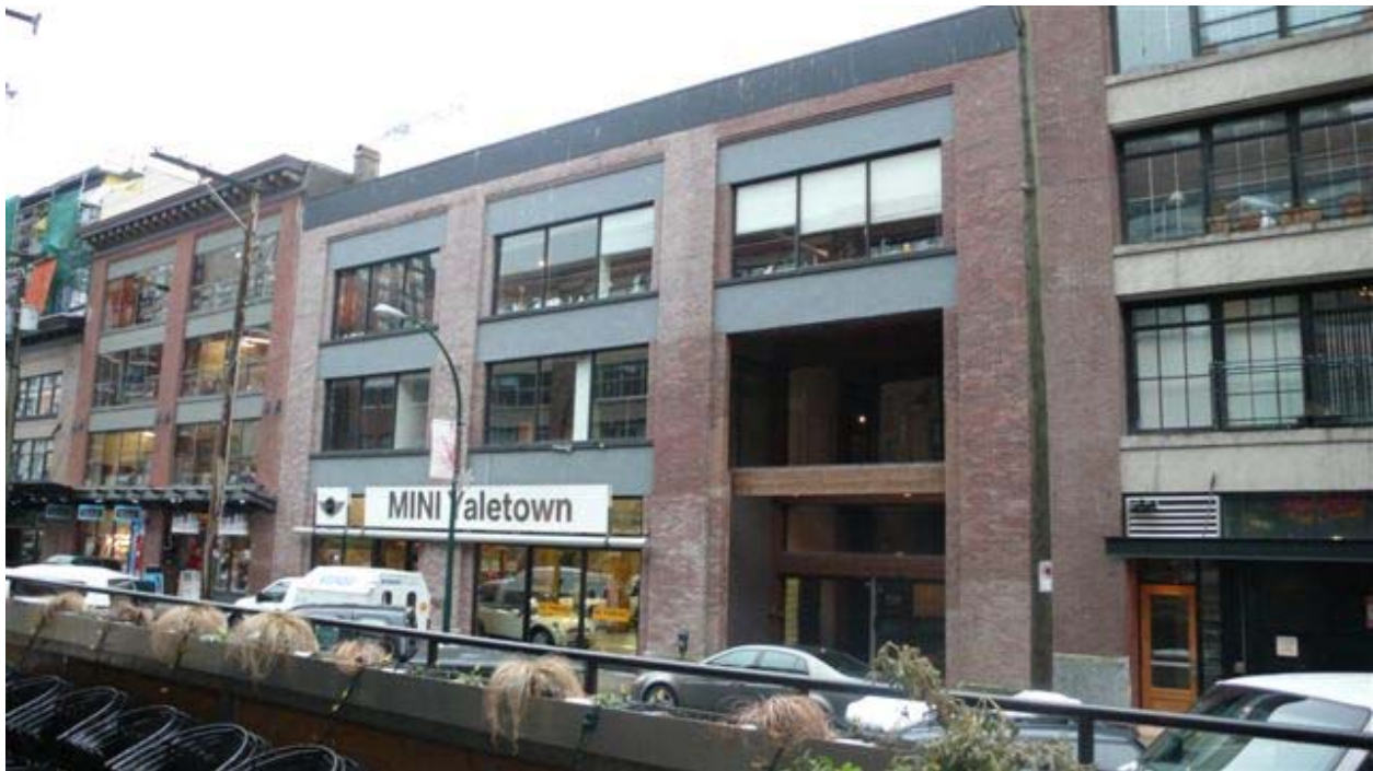
Photo 1: 1132 Hamilton Street - Hamilton Street Side - Existing Condition
