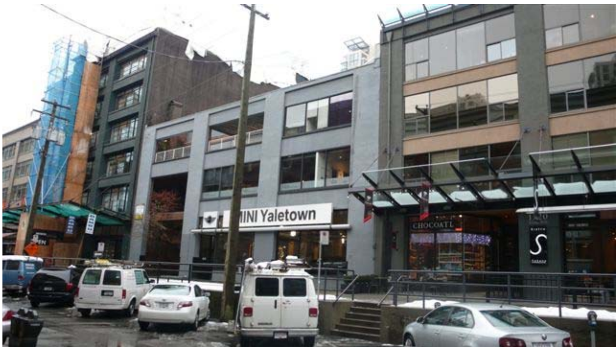
Photo 2: 1132 Hamilton Street - Mainland Street Side - Existing Condition
