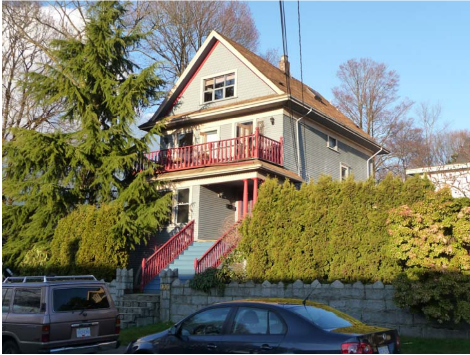
906 Salsbury Drive - Prior to rehabilitation of second floor porch
