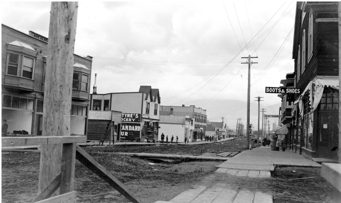
Photo 2: 'The Gow Block' Under Construction, November 1911, Looking North-West
