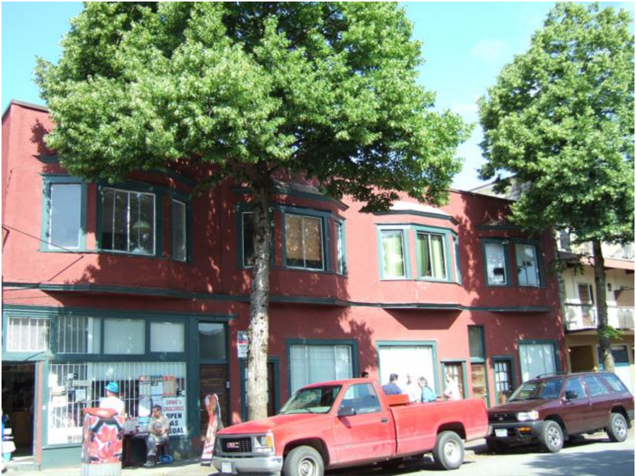
Photo 4: 'The Gow Block' Prior To Recent Renovations and Rehabilitation
